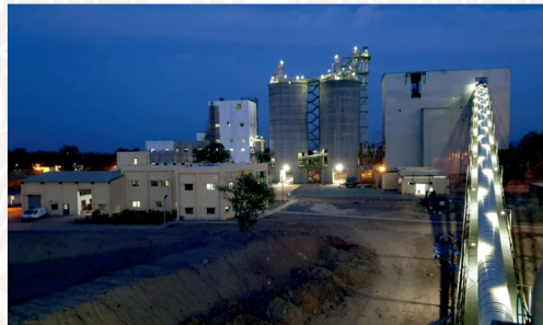
80 TPH CLINKER GRINDING UNIT IN MALI, WEST AFRICA
